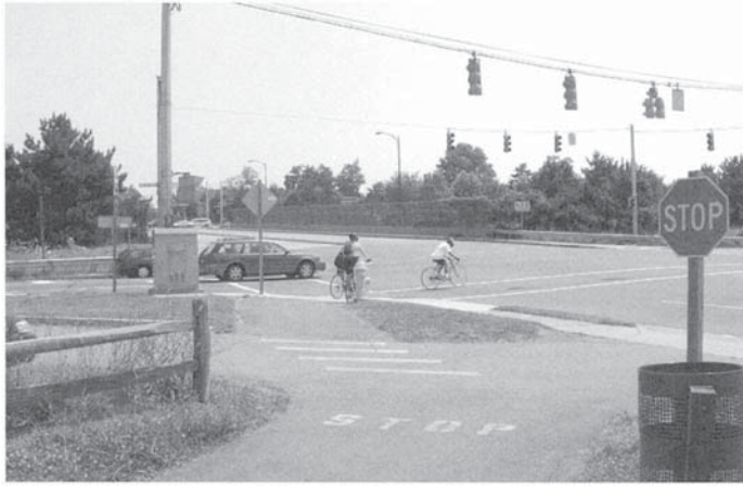
Fig. 12. Crossing a private drive and a busy intersection on the W&OD Trail in Arlington, Virginia.
